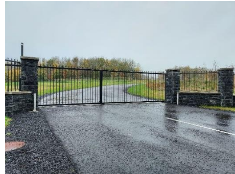
Alternative Incident Control Point – Emergency access road
