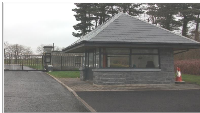
Initial On-Site Co-ordination Point - Gatehouse
